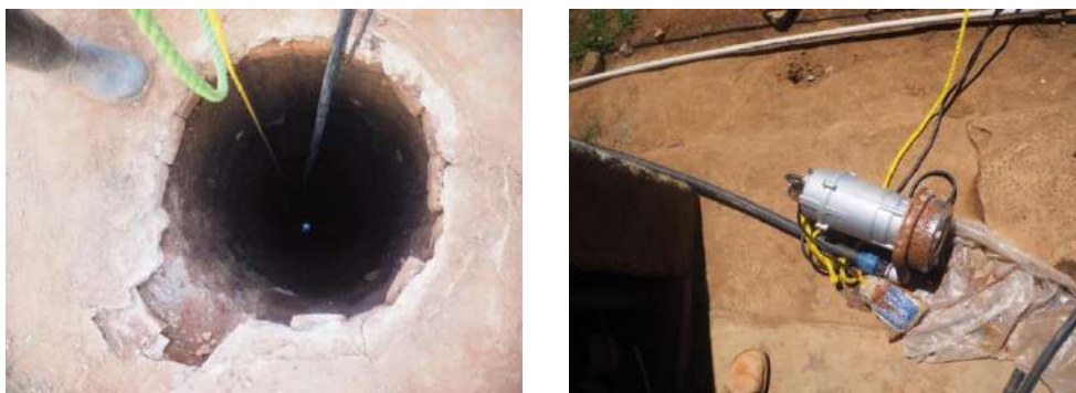
Figure 2: Manual digging inside the well to deepen the well 3 m (left) and the submersible pump used to pump the water out (right).
