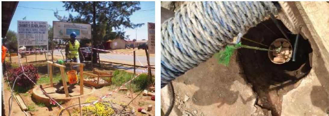
Figure 3: Lining of bricks inside the well to avoid collapsing of the soil.
