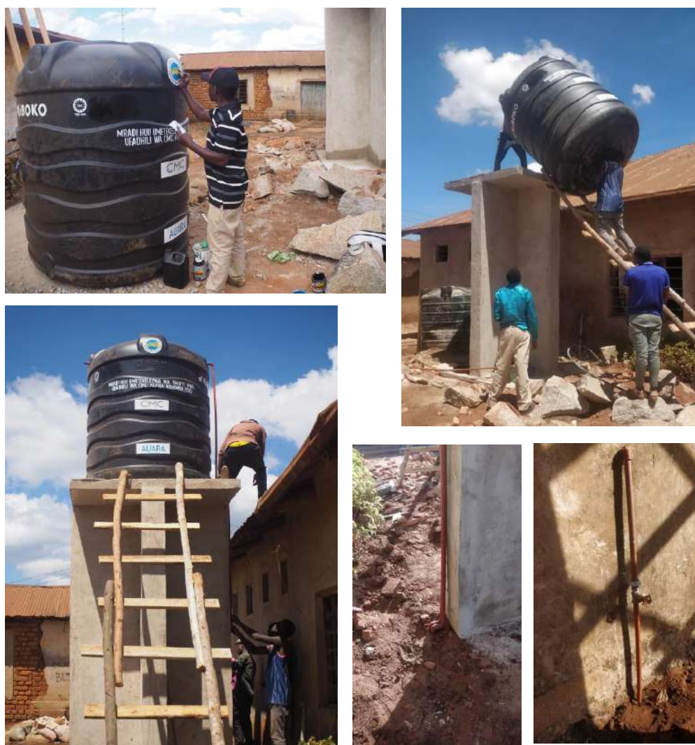
Figure 7: Painting the logos in the storage tank, lifting the tank to the tower and connecting the pipes to the inlet pipe of the dispensary.
