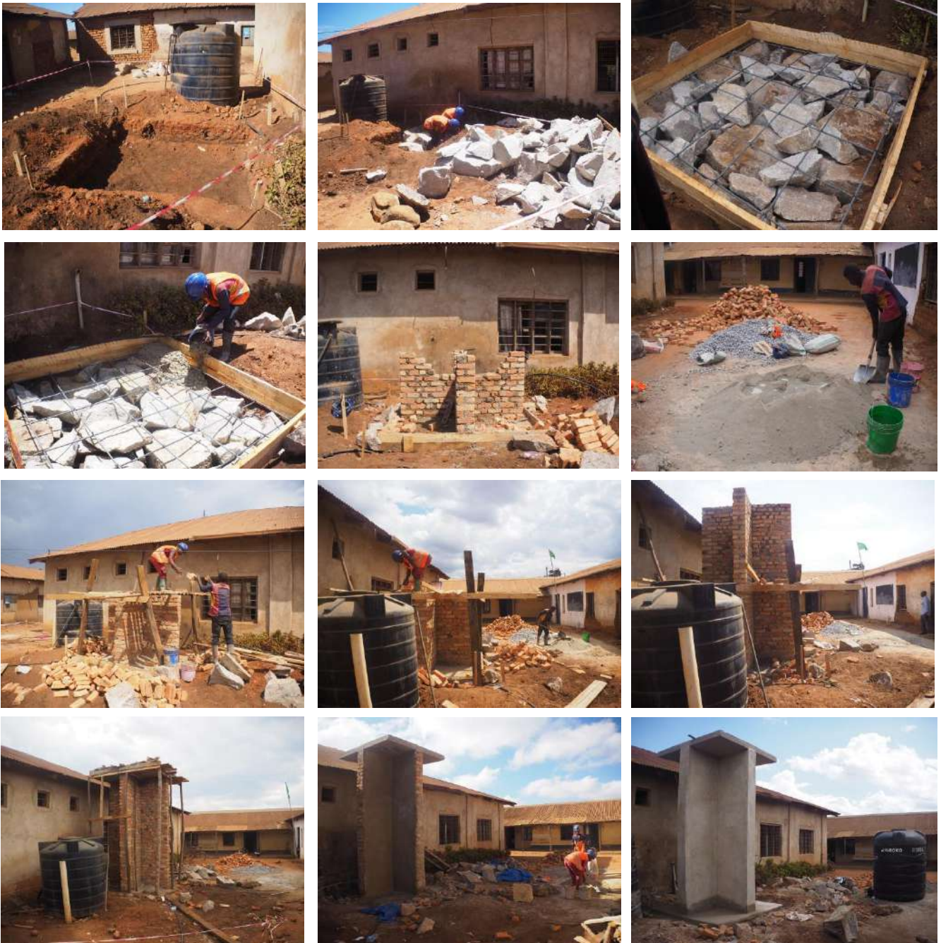
Figure 6: Different steps in the construction of the tank tower.
