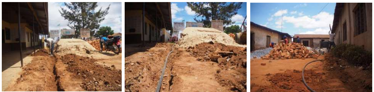
Figure 5: Digging the trenches and installing the connection pipes from the well to the storage tank.
