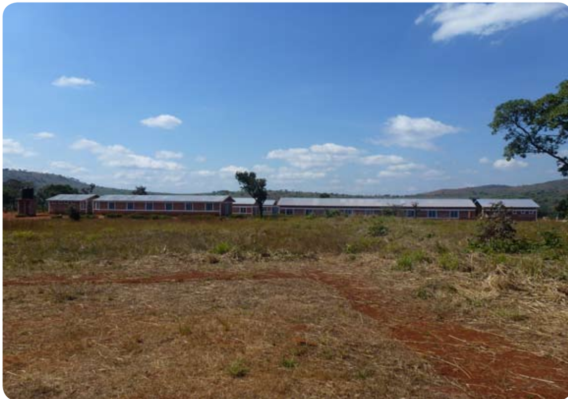
Dormitories in Mundindi Secondary School constructed by SHIPO in collaboration with Mundindi Ward community
