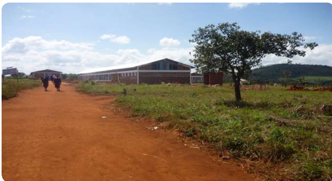
A picture showing a section of dormitories built at Mundindi Secondary School in Ludewa, Njombe region
